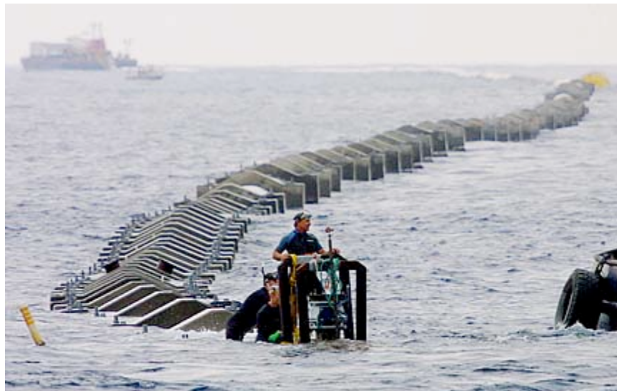
MICHAEL DARDEN / WEST HAWAII TODAY VIA ASSOCIATED PRESS Divers stand on the end of a 9,000-foot, 55-inch diameter pipe floating in the waters near the Natural Energy Lab of Hawaii, north of Kailua-Kona. The pipeline is expected to lead to more development at the Hawaii Ocean Science and Technology Park.
